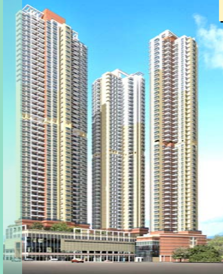
Wanchai Road / Tai Yuen Street Redevelopment
